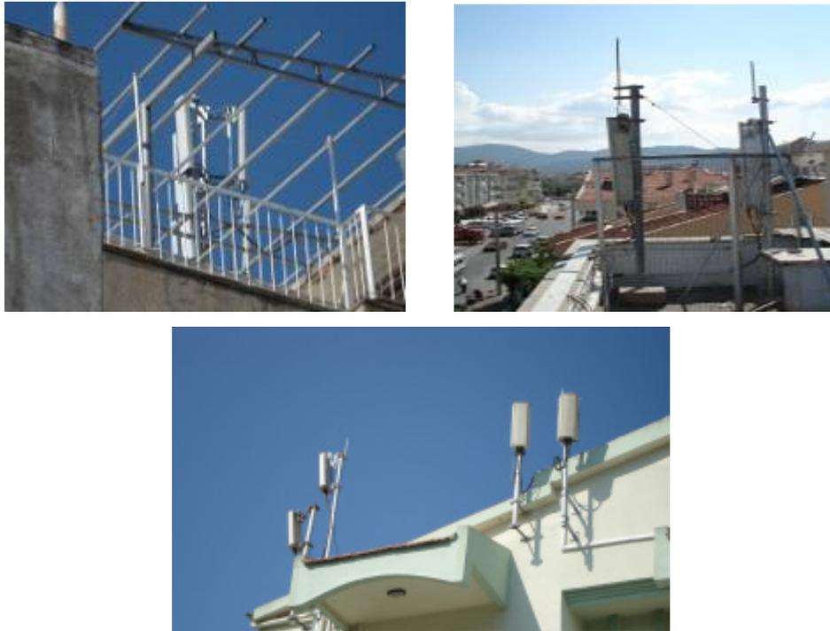
Figure 4.4 Sample roof-top base station installations
