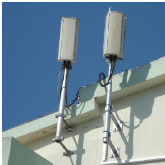
Figure 3.4 Sample wall-mounted RF antennas
